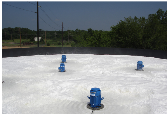
TYPHOON Aerator installation in a paper mill application
