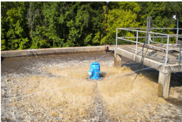
TYPHOON Aerator creates high velocity spray
