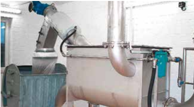
Tank-mounted HUBER Rotary Drum Fine Screen ROTAMAT®...
